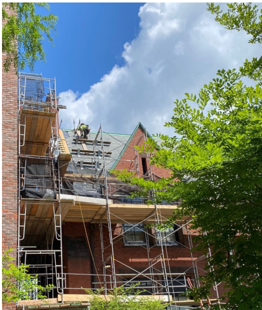
Construction in process Image Courtesy of Genevive Tocci
