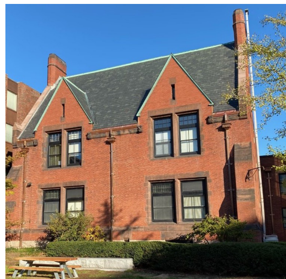
Construction completed Image Courtesy of Genevive Tocci
